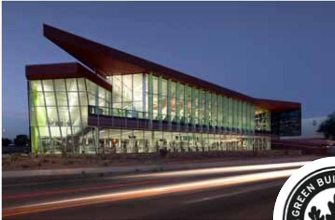
This project is green from the ground up. It was built on the site of a parking lot, which was pulverized and used for stabilizing the footings of the building. On the roof are 346 argon-filled vacuum-tube solar thermal collectors that are expected to harvest almost 2 million kilowatt hours of solar energy per year.
