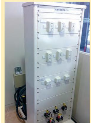
Load connection panel for experiments
