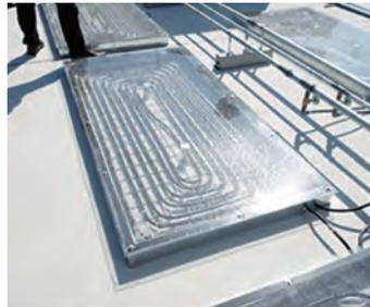
Heat radiation piping unit under the slab
