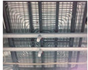
Thermal Storage Radiation Air-conditioning System using underground heat
